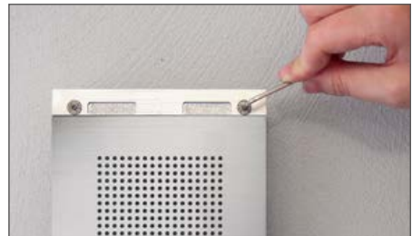
3 Connect and fix the door intercom station
